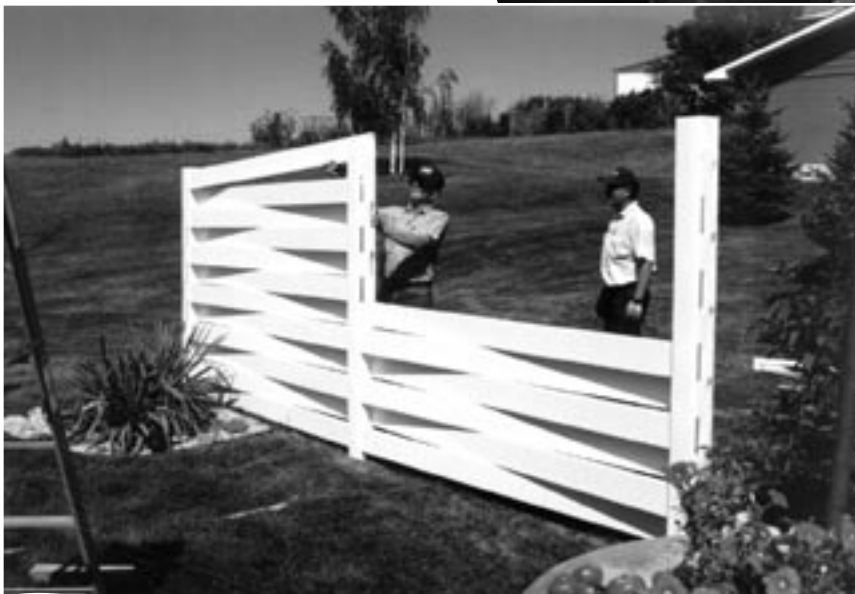
Sections or rails are added until the fence is complete.
