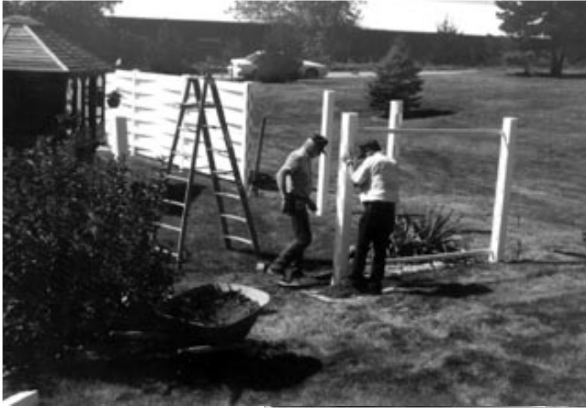
Posts are set for the entire installation.
