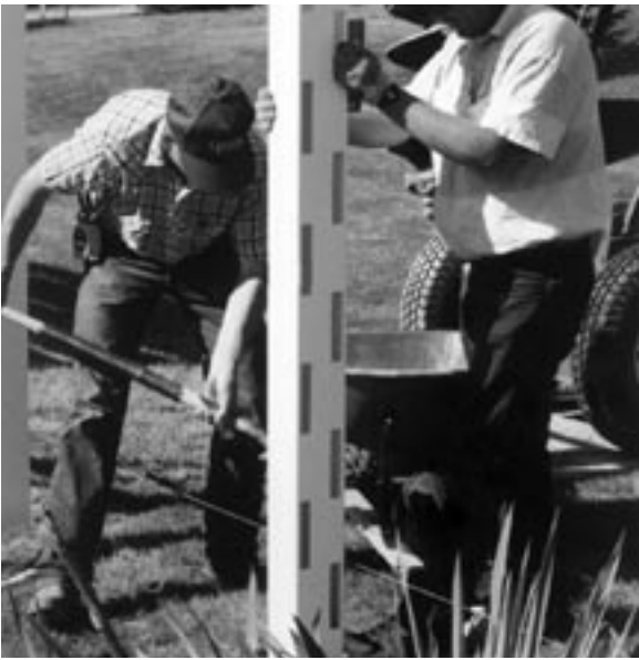
Post placement is important, using a stringline and level to assure vertical alignment.
