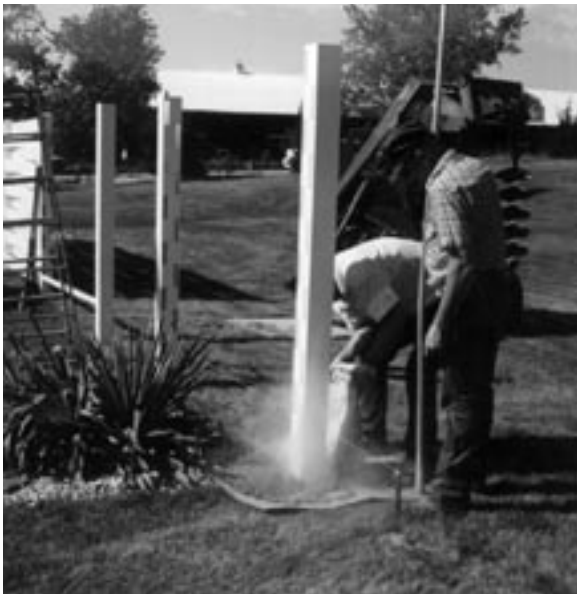
Once the post is aligned, cement or a cement-water mix will make it permanent.
